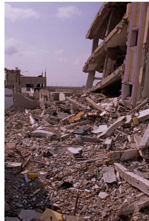
Destructed homes in Rafah, Gaza
